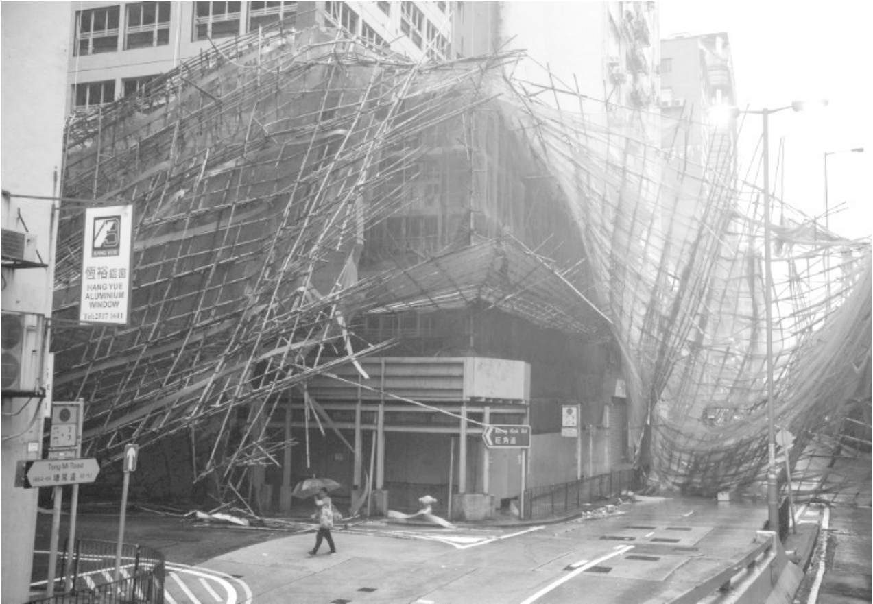
Typhoon Mangkhut stripped traditional bamboo scaffolding from constructions sites across Hong Kong
